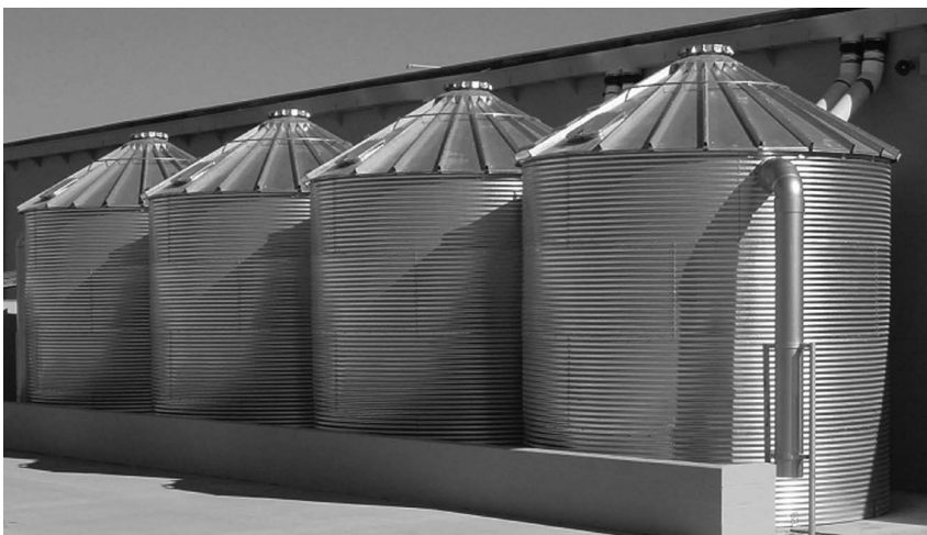
Industrial tanks such as these can store hundreds or thousands of gallons of rainwater that has been collected from rooftops for later use.
